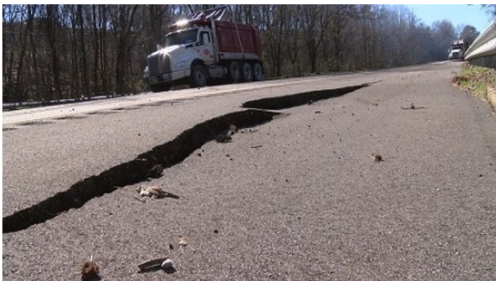
Severe cracks in Hwy 231 caused by a local landslide. Source: ABC WAAY 31. March 06, 2020
